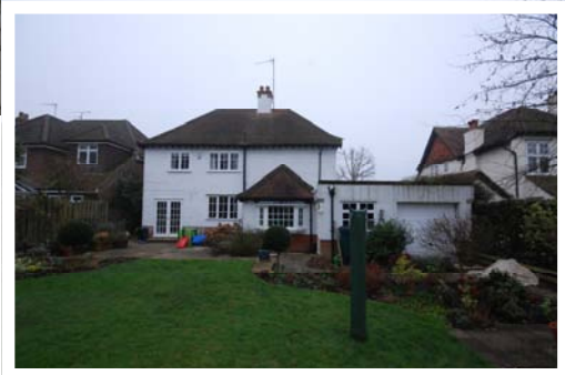
Original rear elevation
